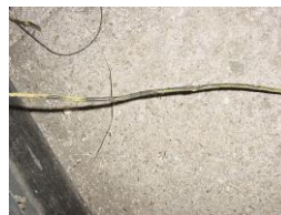
Above: Burst tube following overheated cable
